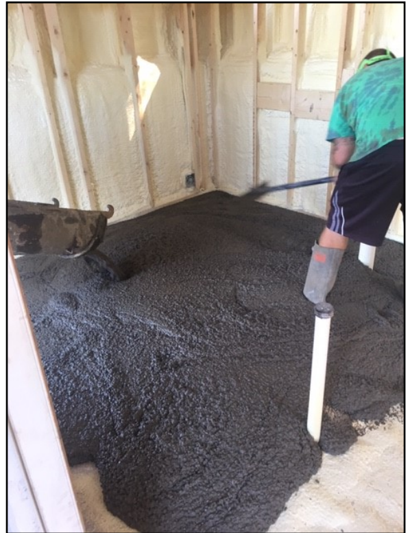
Interior View ...floor going in!
