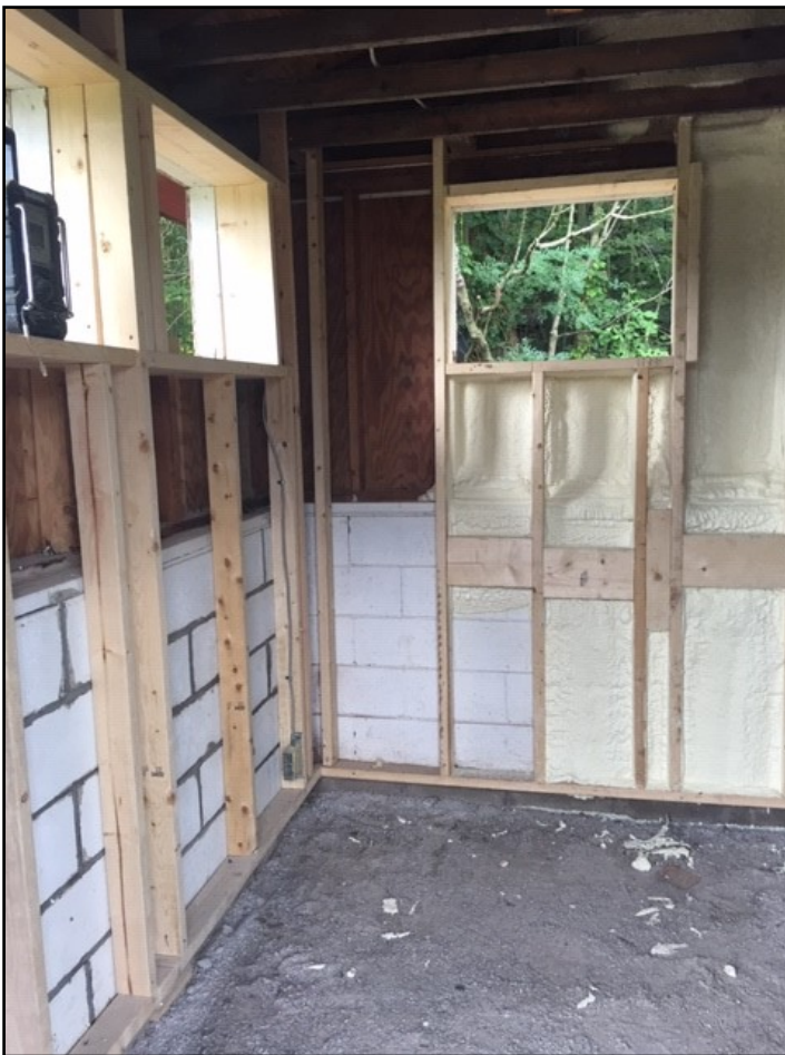
Interior View ... walls under construction!
